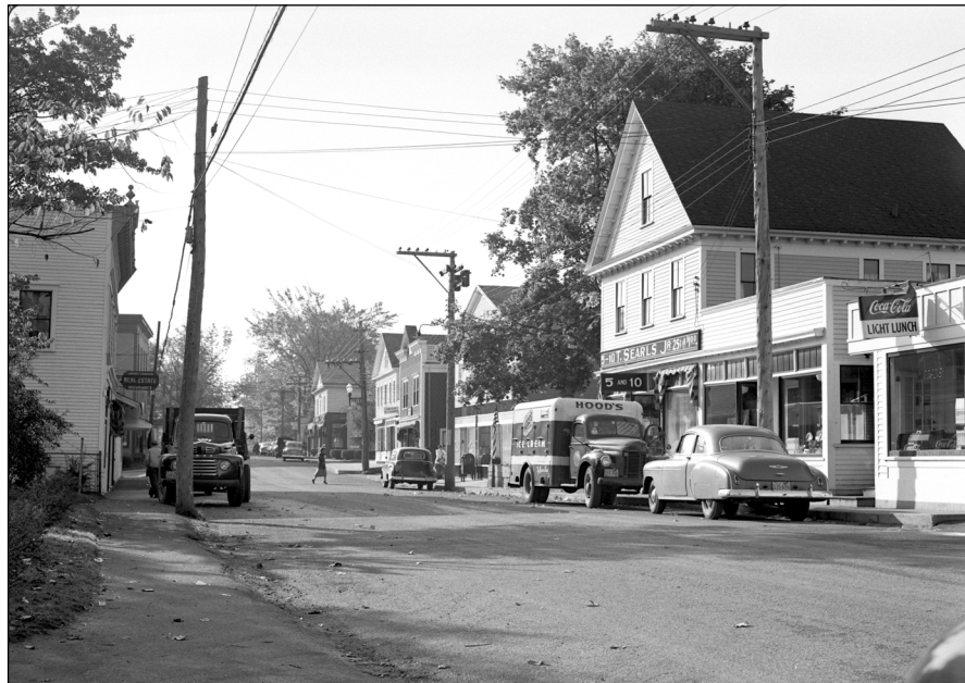
View South on Main Street from Pemetic School Sidewalk - October 20, 1951 Photograph by W.H. Ballard Number 7858 - The Southwest Harbor Public Library Collection of Photographs
