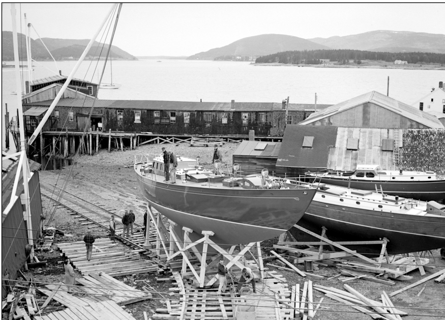
The Henry R. Hinckley Company Yawl, "Venturer" Built for Harry Garner Haskell Jr. - On the Ways - May 14, 1956 She was the largest wooden boat built by the Hinckley Company Photograph by W.H. Ballard Number 12061 - The Southwest Harbor Public Library Collection of Photographs
